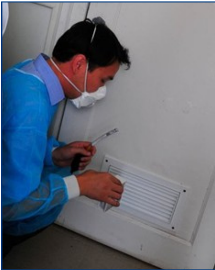
Figure 22. Technician using both a commercial smoke generating tube and a swinging vane anemometer to verify that air is moving into the room. In addition, the anemometer can be used to measure the speed of the air coming into the room. Knowing the area of the grille and the speed of the air, the volumetric airflow rate into the room can be calculated.
