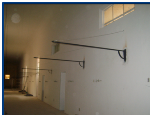
Figure 6. Hospital Patient Ward after renovation
