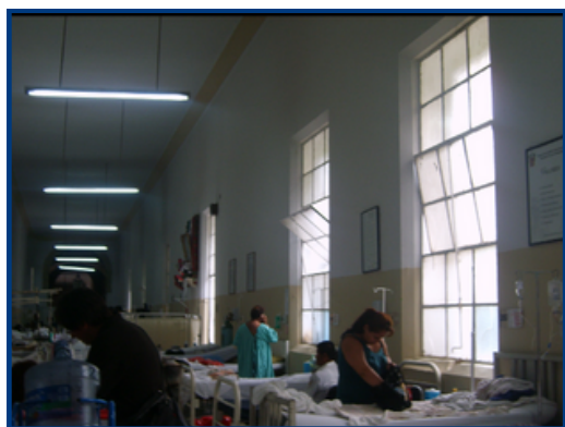
Figure 5. Hospital Patient Ward before renovation
