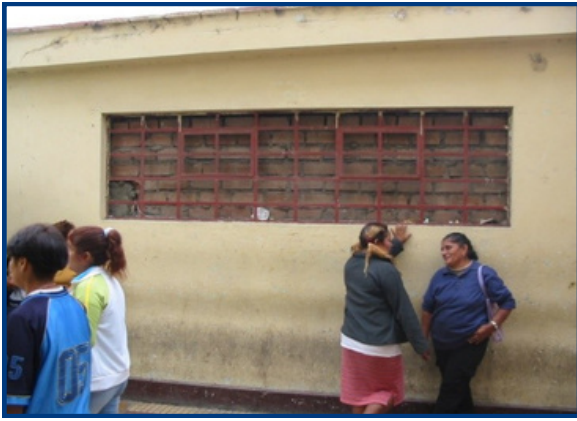
Figure 27. An example of a renovation where a window was bricked up.
