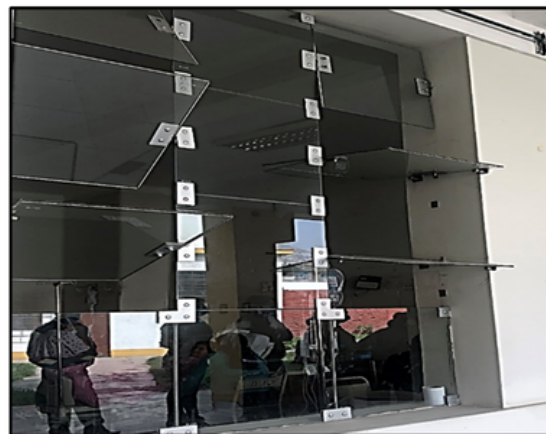
Figure 18. Naturally ventilated waiting room after renovation of space.
